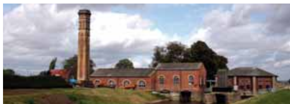
Lade Bank Pumping Station
